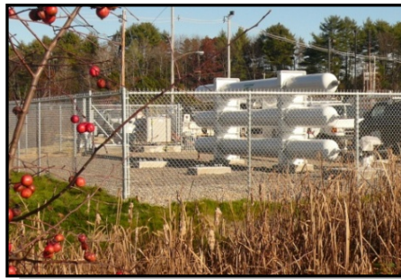
Phase II CNG Fuel Station – fall 2010
