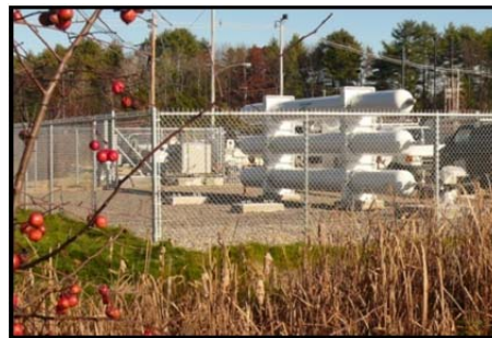
Phase II CNG Fuel Station – fall 2010
