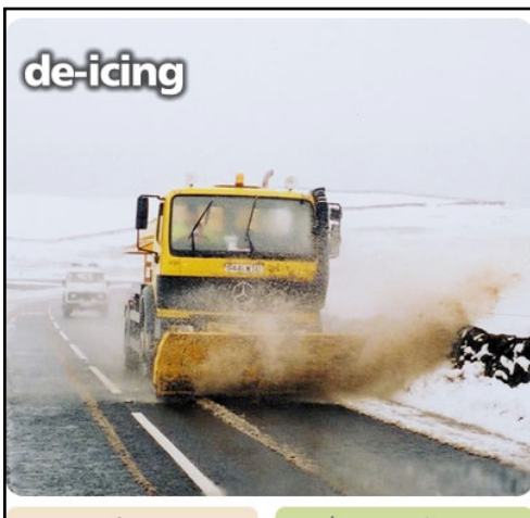
Deicing Treatment on a roadway
